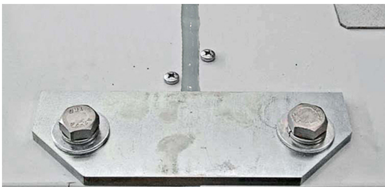
Figure 38 – Roof joint
