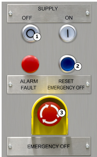
Figure 86 – Detail of local control panel on the COU
